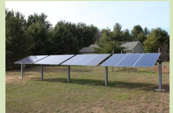
3.72 KW Adjustable Ground Mount Solar Array at the home of Craig and Vicki Olsen
